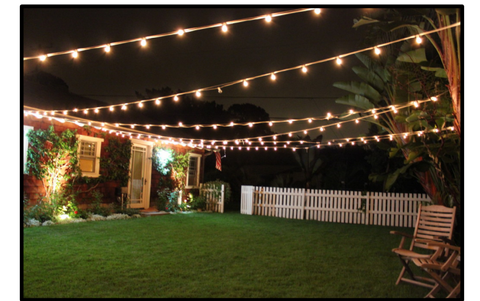
Overhead String Lighting
